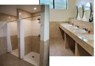
The Habilitat Construction Crew did an amazing job of renovating the female bathroom this year. Using the funds we were granted from the Harry & Jeanette Weinberg Foundation, they completely gutted the entire room, made major repairs, replaced all of the fixtures and laid new tile. The renovation improved the bathroom's functionality and gave our female residents much more space.
